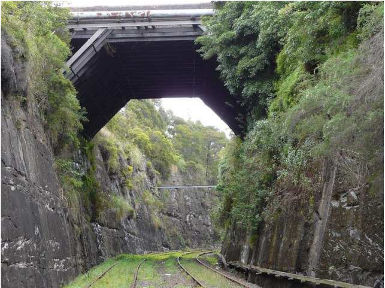
Illustration 9: Balmain Road Overpass - looking west
