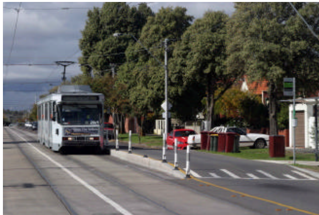
Figure 5: “Vienna” platform in Melbourne showing retained driveway access to adjacent property
