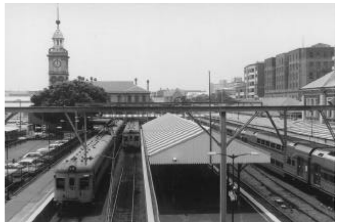
Newcastle Railway Station has the added benefit of being conveniently located near the CBD and a short walk from the State Transit bus and Stockton ferry terminals
